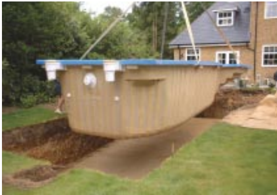
The pool is dropped directly into the hole - simple!
