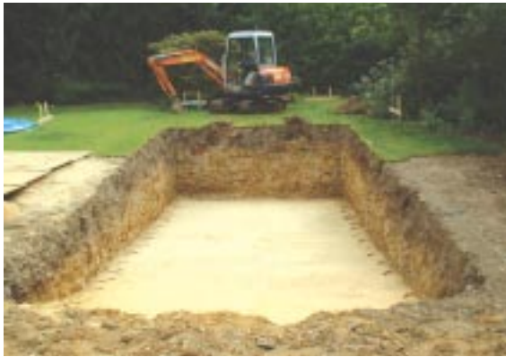
The hole excavated and base prepared ready for the pool.
