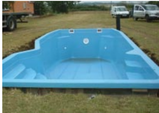
Back fill and add water, the pool is ready to go!!
